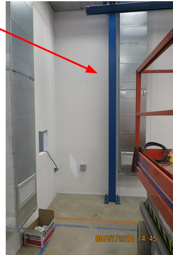
Photo of SW Corner
